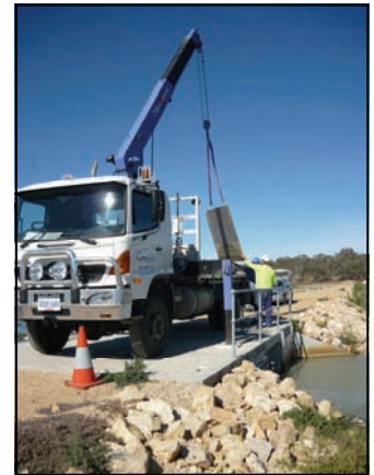
above: Sluice Gate Comes Out
